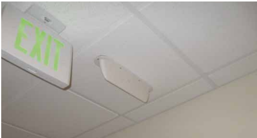
A typical VHF antenna often used in VHF DAS systems
