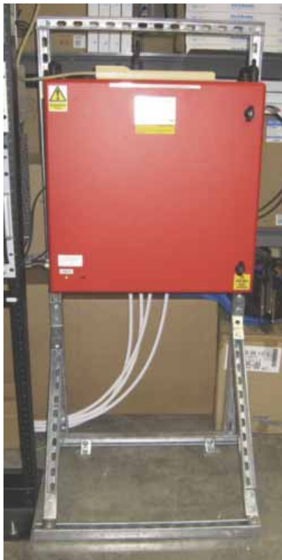
A bidirectional amplifier (BDA) is used in a DAS deployment.
